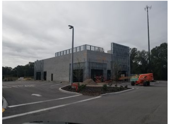
Building During Construction Dec 4 2018
