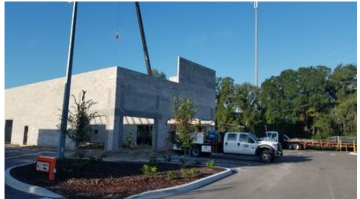
Building During Construction Sept 6, 2018
