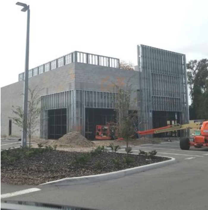
MDI Bldg 2 Under Construction
